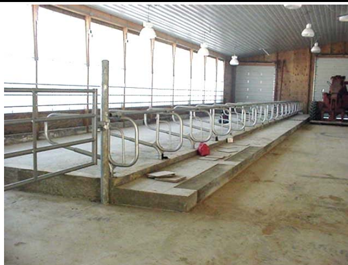
The new research facility (under construction) is located near the holding area of the new barn. The sixteen tie stalls will allow our research staff to conduct research requiring individual dry matter intake measurements.
